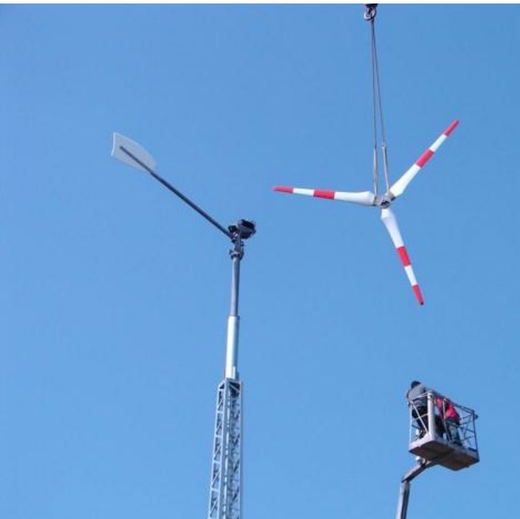
Picture 7: Pre-mounted rotor
