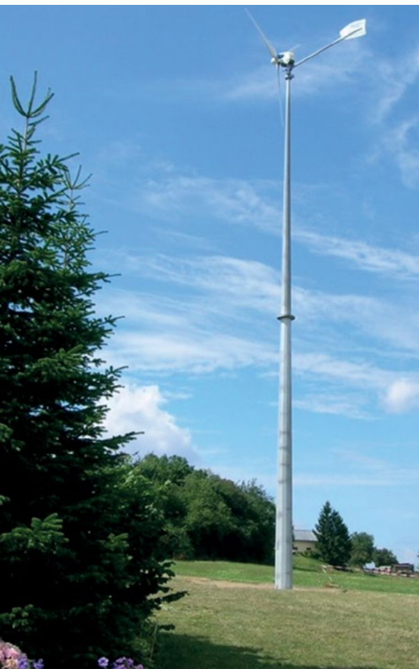
Picture 1: Freestanding mast readily mounted
