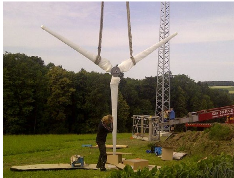
Picture 7: Pre-mounted rotor
